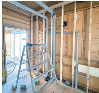
The drain lines coming from the washroom loads and the load from seven hotel suites running to the Sanicubic 2VX.
