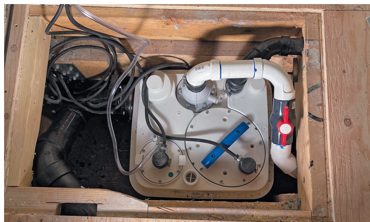
The Sanicubic 1 positioned in a small space under the floating home's wooden floorboard. AR Plumbing owner and CEO Adelsio Rodas and his team used two of the four inlets on the Sanicubic 1.
