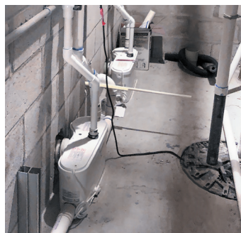
Sanibest Pro grinder units installed to discharge the wastewater from three toilets and a urinal. The two toilets in the women's restroom are each connected to a Sanibest Pro unit.
