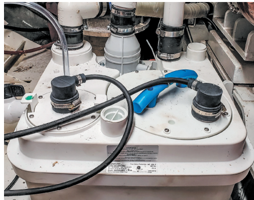
Inside the RV MANTA's mechanical room, showing the Sanicubic 1 and the 1.5-inch PVC piping to two of the Sanicubic 1 's four input ports.
