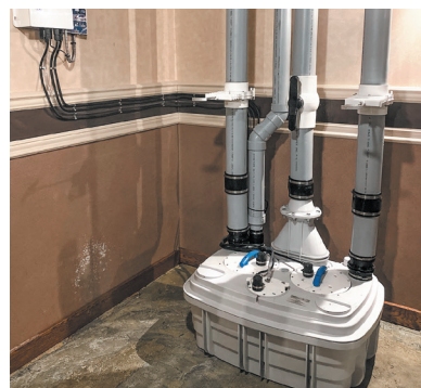
Albanese installed the Sanicubic 2VX in the hotel's basement. The 4-inch discharge pipe runs from the top of the Sanicubic 2VX 10.5 feet vertically and 25 feet horizontally before tying into the existing drain line.
