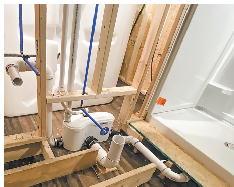
Bathroom 1: Showing the shower's drain line connected to the Sanigrind Pro's 2-inch inlet.
