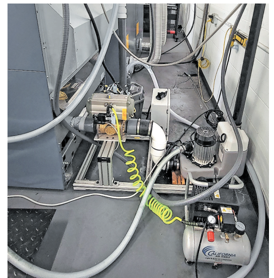
The pretreat coming from the washing machines flows into the Sanicom unit. The Sanicom pumps the liquid five feet via hose into the reuse tank connected to the washing machine.
