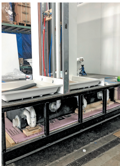
View of the plumbing set up below the trailer's finished floor frame.
