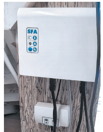
The control panel of the Sanicubic 1 has a visual and audible alarm system (including a 15' wire).
