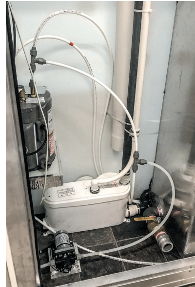
Sanibest Pro installed in portable washroom unit.
