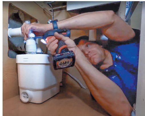
Dane Perkins, Co-owner and Project Manager of GMH Construction is installing the newly Sanivite drain pump.
