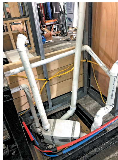
The Sanishower drain pump is small enough to fit comfortably under a raised shower base.
