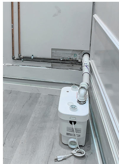
The 1.5-inch rigid pipe connected to an existing PVC discharge pipe running to the building’s sewage access.
