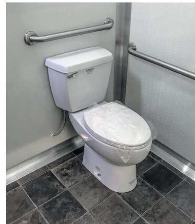
Saniflo's elongated rear discharge toilet is ADA compliant which facilitates the installation of all the bathrooms.
