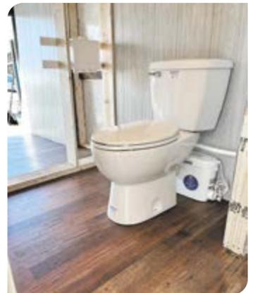
The wastewater from the toilet drains into the pump unit, which incorporates a grinder system to quickly reduce the incoming effluent before discharging it through small-diameter plastic piping up to 25 feet vertically or 150 feet horizontally to a sewer or septic system — or, in the case of SOLT, to a storage tank.
