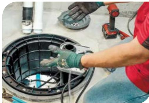
The retrofit pump kit seamlessly fits into existing 24-inch basins from leading manufacturers, eliminating the need for extensive plumbing modifications.
