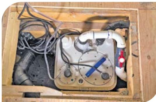
The Sanicubic 1 positioned in a small space under the floating home's wooden floorboard. AR Plumbing owner and CEO Adelso Rodas and his team used two of the four inlets on the Sanicubic 1.
