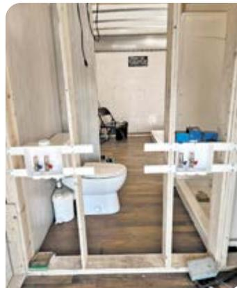
The **Sanibest Pro** combines a rear-discharge toilet with a 1-horsepower pump system that is usually situated on the floor behind the fixture (and sometimes, for aesthetic reasons, concealed inside the wall behind the toilet). The system can be used to install a complete bathroom, including a toilet, sink, tub, and/or shower.
