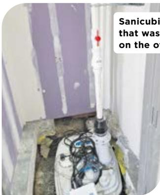
Sanicubic 2VX was installed in a closet that was created specifically for the pump on the other side of the bathroom.
