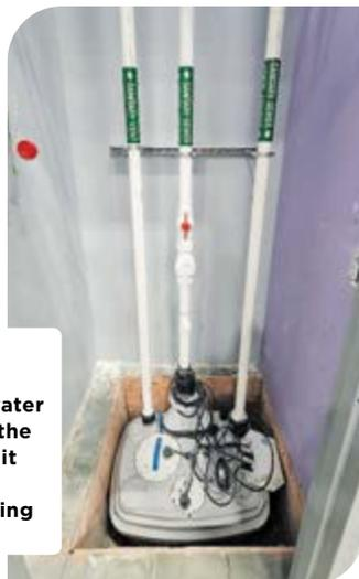
The second Sanicubic 2VX was installed for two side-by-side restrooms, also receiving wastewater from the first Sanicubic 2VX. All the wastewater within this second unit discharges into the conventional plumbing system of the pre-existing restrooms.
