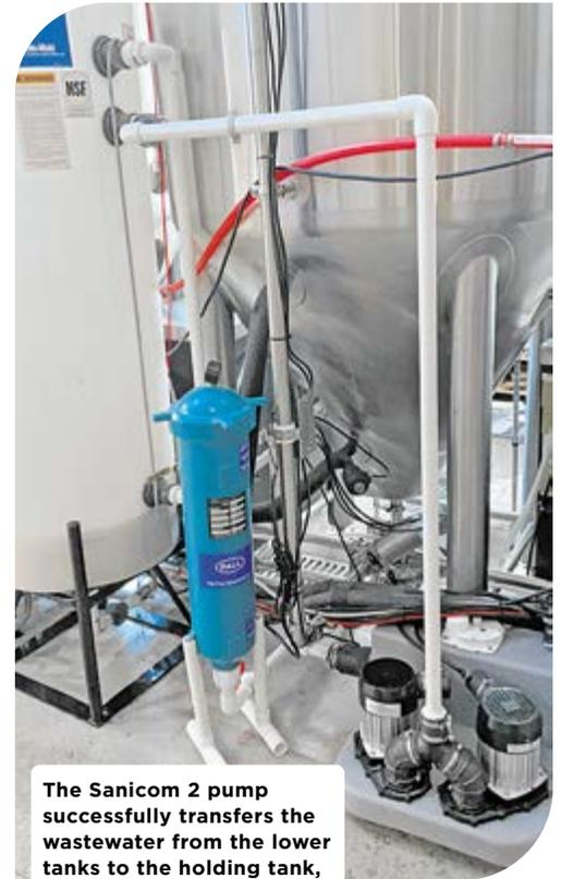
The Sanicom 2 pump successfully transfers the wastewater from the lower tanks to the holding tank, enabling the brewery to comply with the town's regulations.
