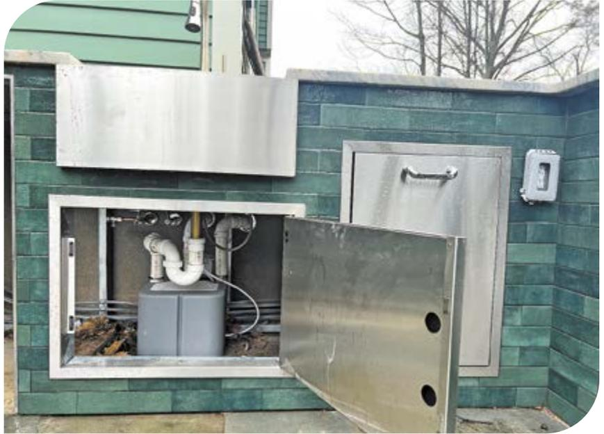
You can easily service the Saniswift Pro without removing any piping. The top cover has two removable screws, providing ready access to all electrical components inside. The pump motor can then be quickly lifted from within to remove any foreign objects in the impeller.
